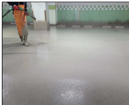
Aquakeeper applied (elastic mortar)
