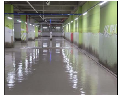
Aquakeeper applied (elastic mortar)
